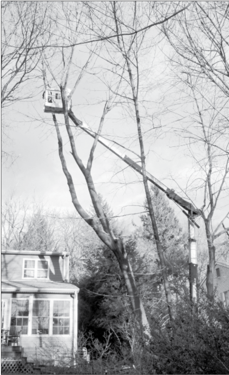
Joe Ross removing a hazard tree using a Teupen 75' self propelled tracked lift.
