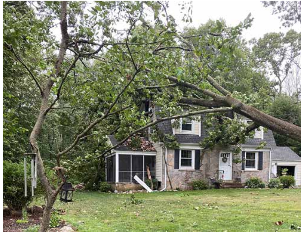
Storm damage to an Orange home
