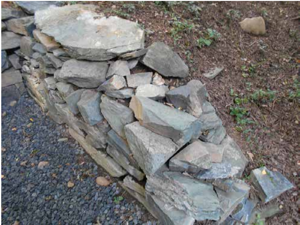
The foundation wall
