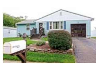
Hamden, 255 Hepburn Road $239,900
